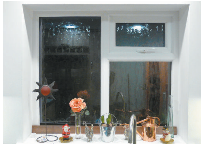
Only a small part of this window can be opened for ventilation, making it difficult for an intruder to enter.
